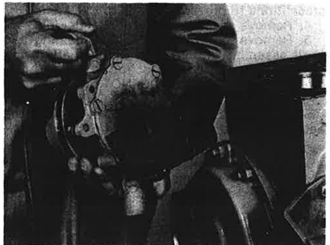
Removing Water Pump
